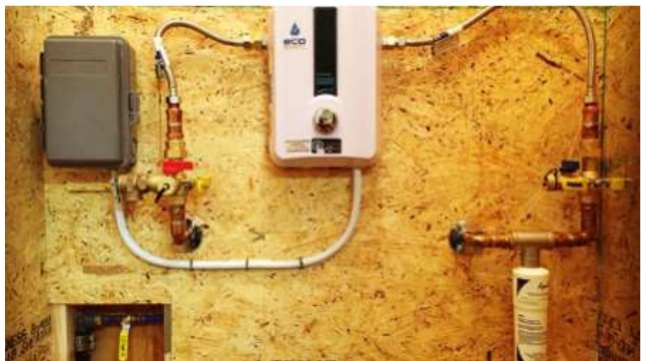
Instantaneous hot-water heater
