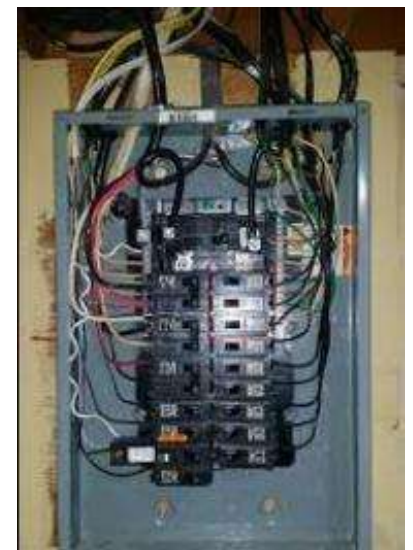
AFCI "breaker" used in a breaker board
