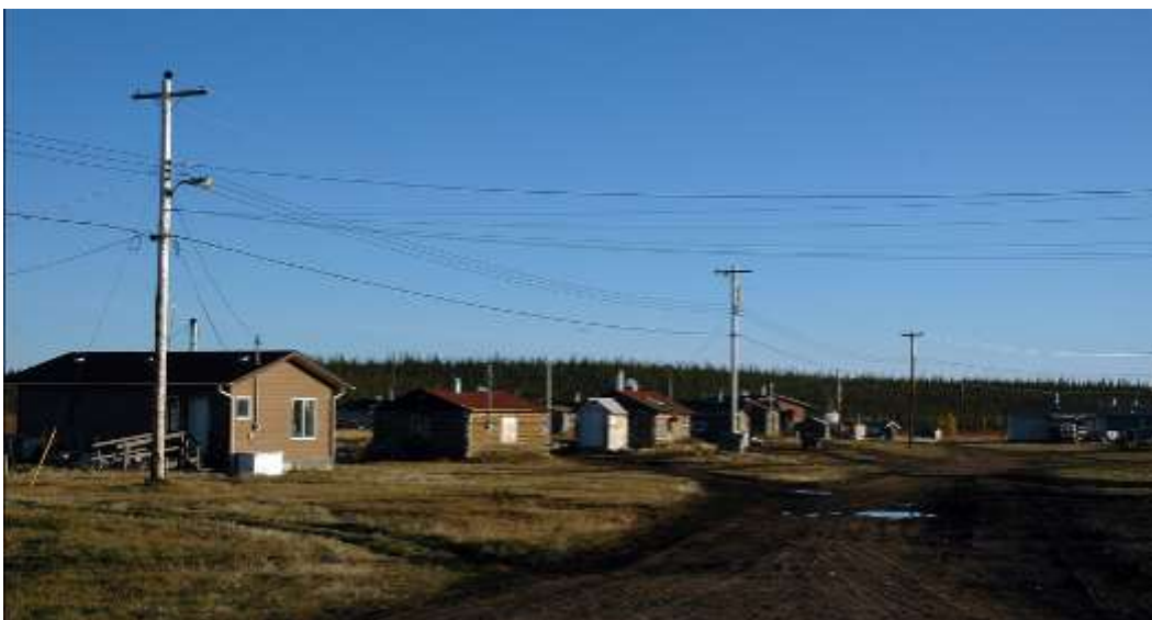
Power-pole installations within a community
