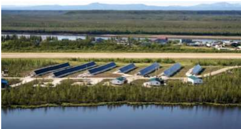
Solar farm installation
