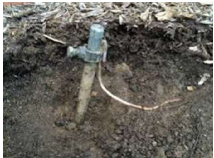
Typical ground installation
