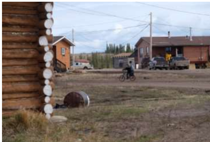
Power-pole installations in a community
