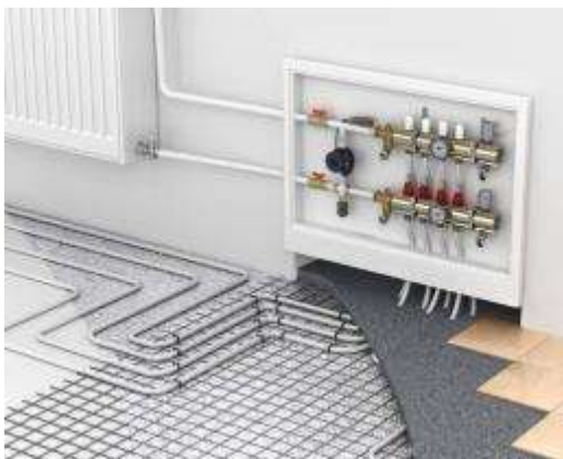
Hydronic radiant-heat flooring
