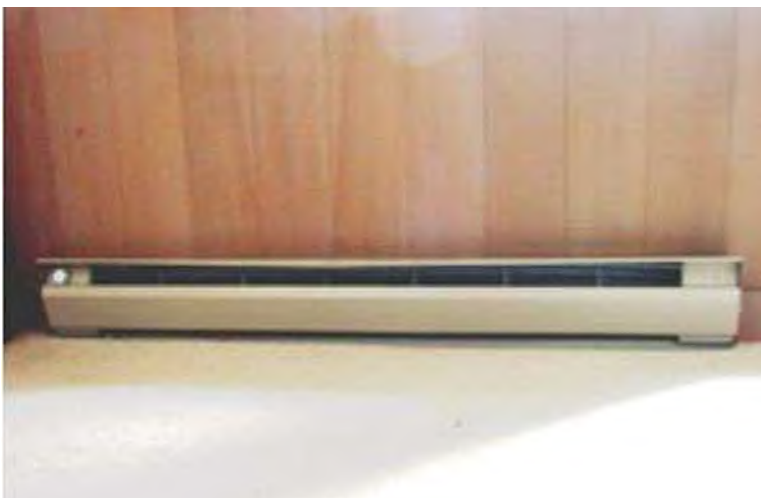
A typical electric baseboard heater that would be located in each room of a house
