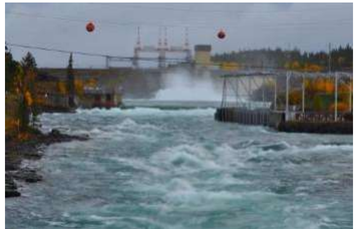
The hydroelectric generation dam in Whitehorse, Yukon
