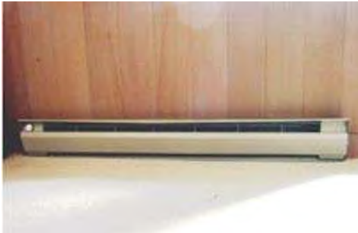
A typical electric baseboard heater that would be located in each room of a house.
