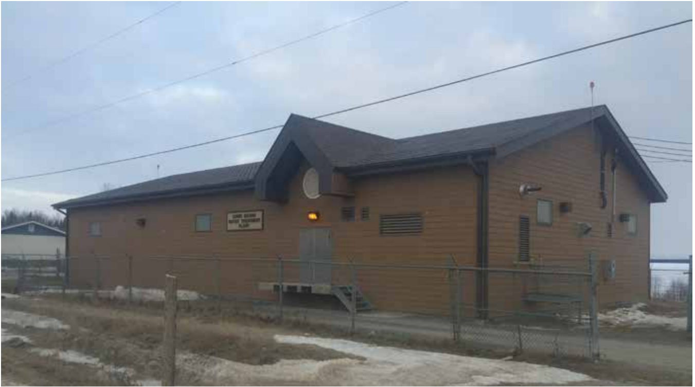
Figure 31 : Water Treatment Plant.
