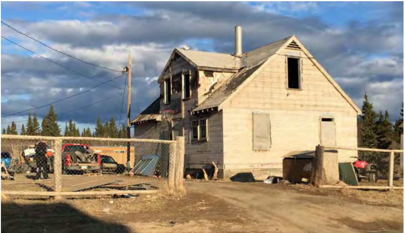
Figure 49 : The oldest known house in BCN.
