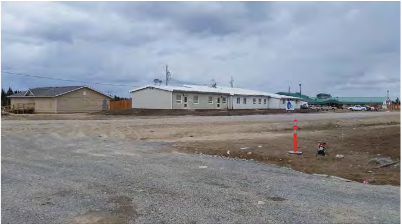
Figure 28 : University College of the north with portable classrooms and 1972 Memorial High in background.
