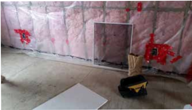
Figure 81 : new split-level home crawlspace walls
