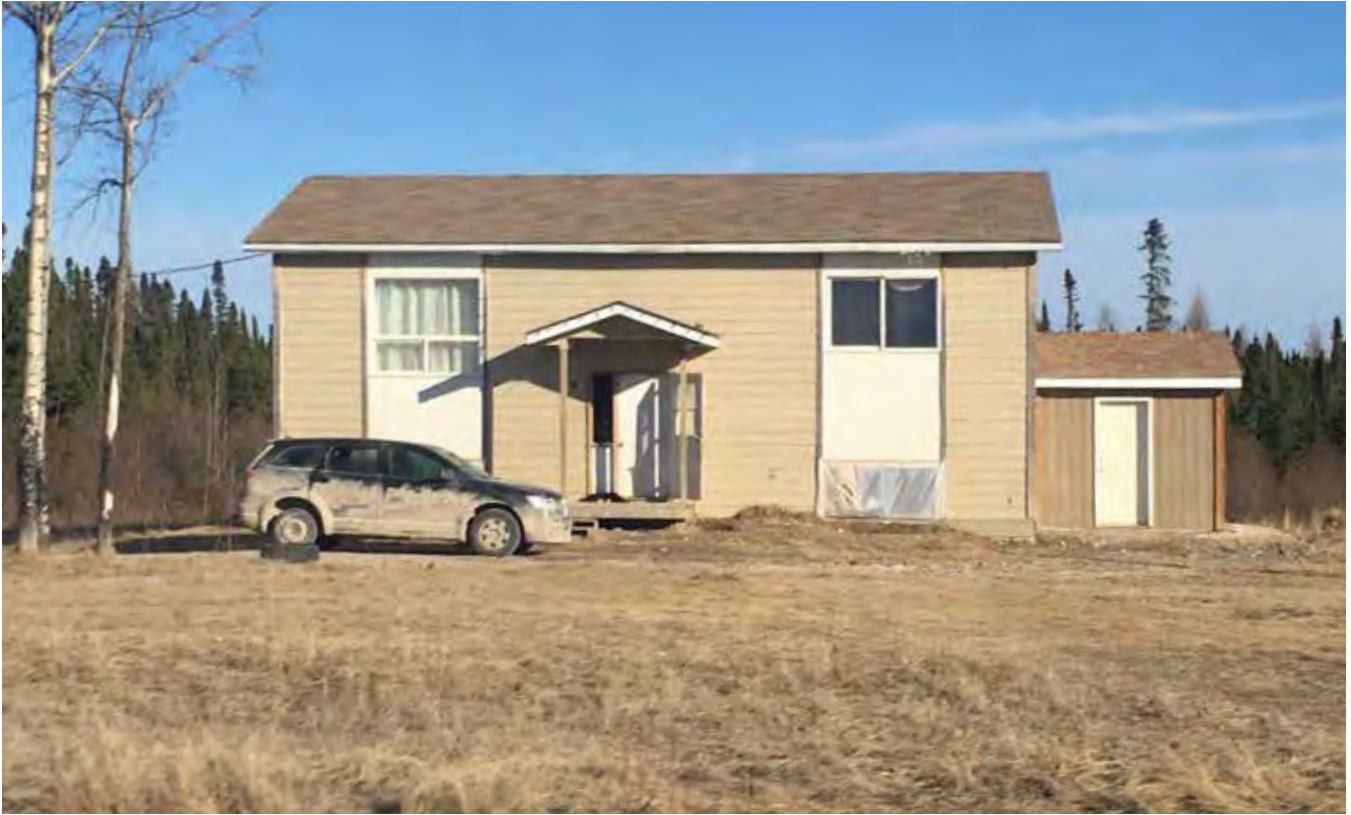
Figure 64 : split-level with broken windows and add-on water tank room
