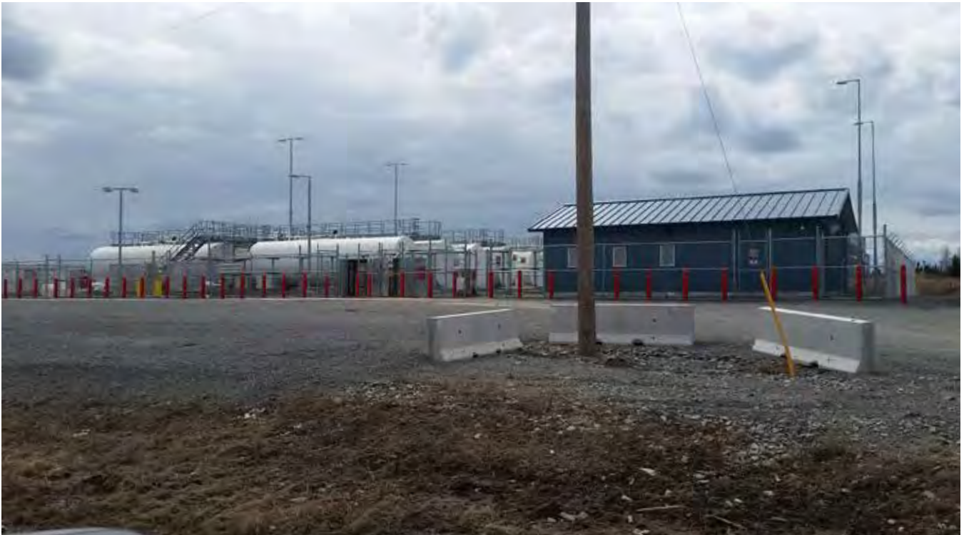
Figure 27 : Public works fuel storage area.
