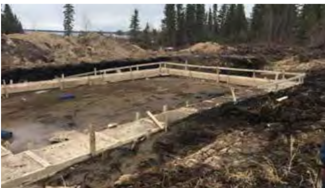
Figure 78 : abandoned concrete strip footings
