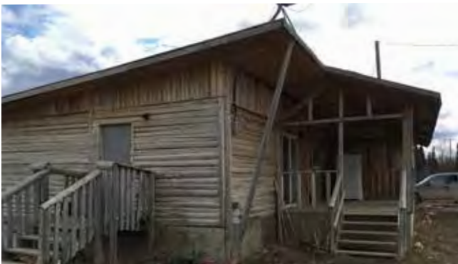
Figure 84 : locally-sourced small-scale timber structure
