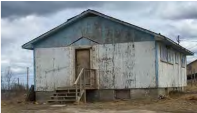
Figure 76 : older bungalow on concrete block foundation
