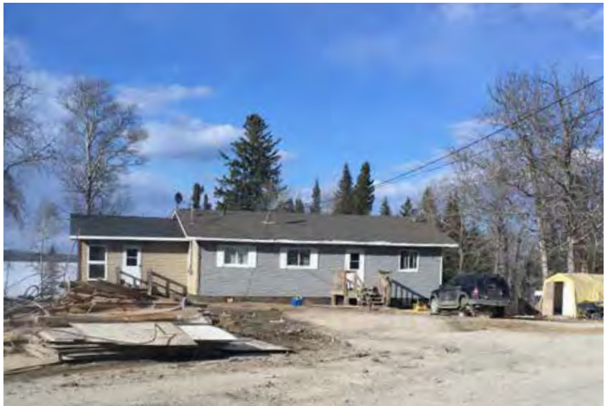
Figure 54 : split-level with broken windows and add-on water tank room
