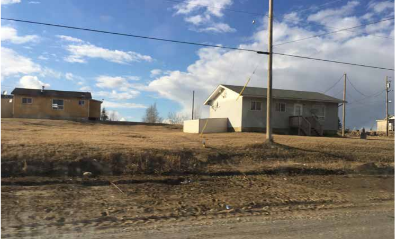
Figure 58 : bungalows with add-on water tank rooms
