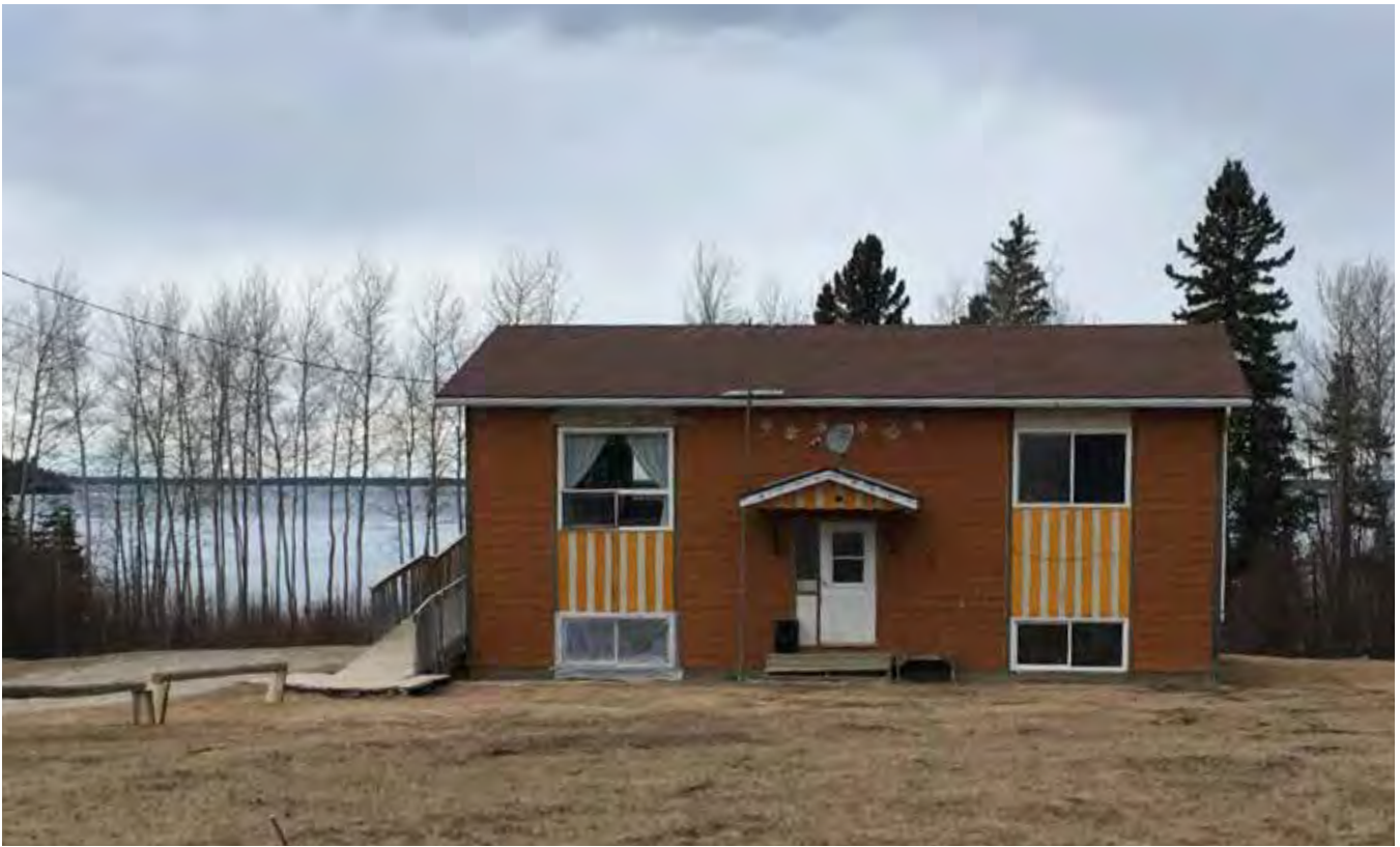
Figure 63 : split-level with add-on water tank room
