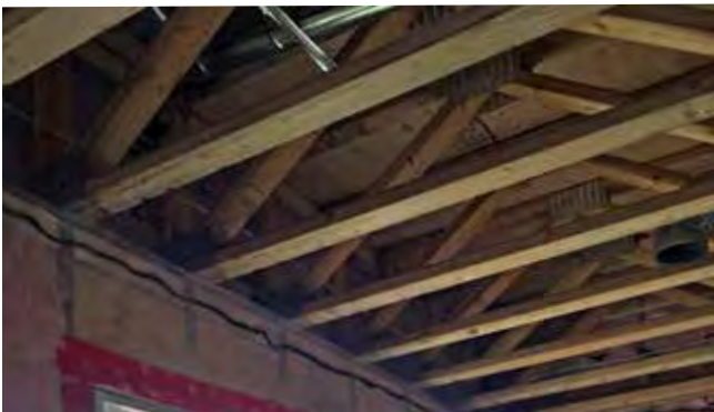
Figure 82 : new split-level home main floor trusses
