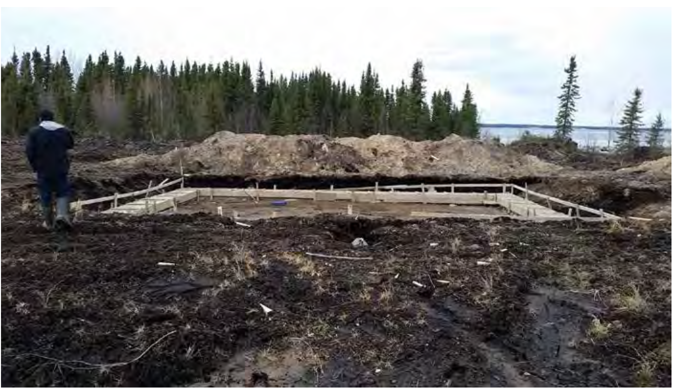
Figure 55 : abandoned concrete footings in southern neighbourhood of BCN
