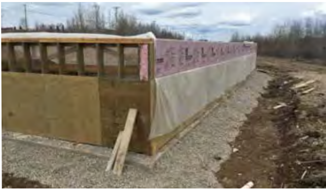
Figure 75 : new split-level home under construction
